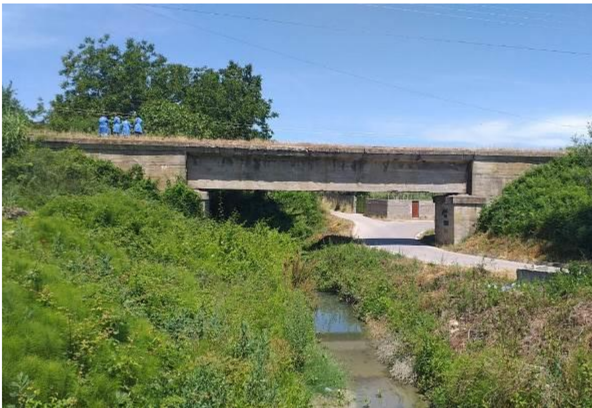
Figure 2.12_Nenkalim ne km 22+240
